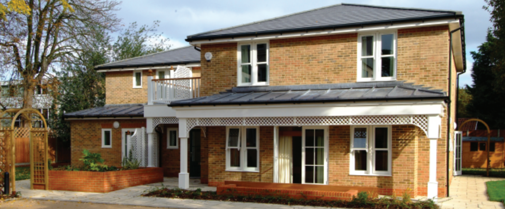
This care home in Richmond, Surrey houses eight adults with learning disabilities. It was designed by local firm HTP Architecture, which also acted as project manager
